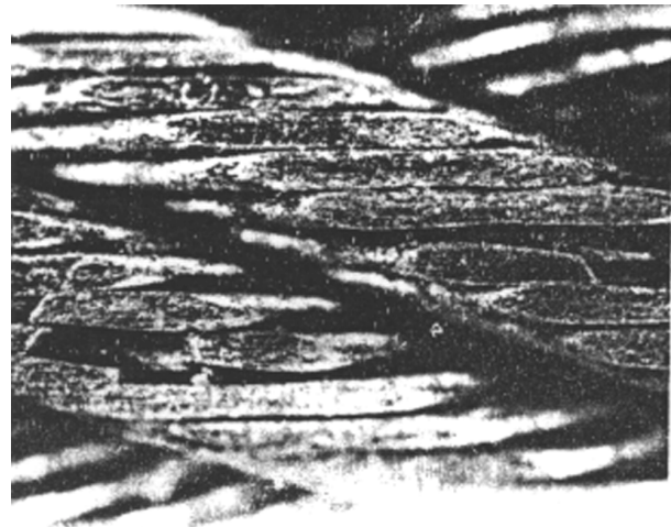
FIGURE 7-18. Worn cable (replacement necessary).
