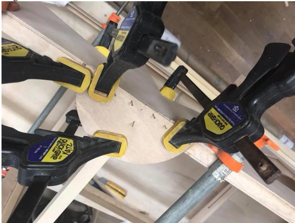
Figure 16: Holding gusset in place for nail installation
