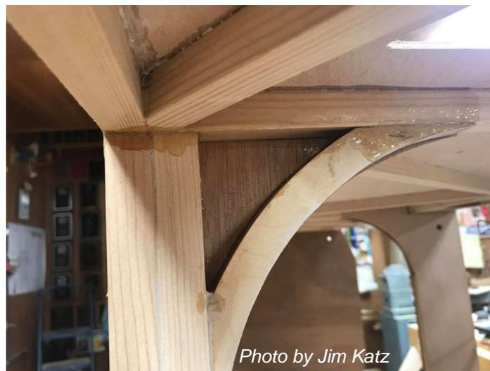
Figure 38: Varnish inside the Corner Bows
